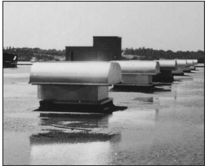
Hooded Propeller Roof Ventilator
