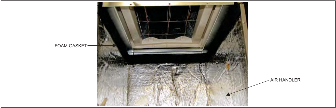
FIGURE 4: Gasket Location
