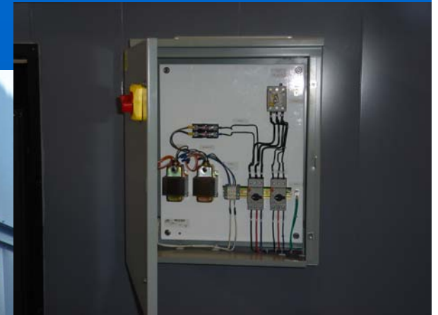
Single Point Electrical Connection
